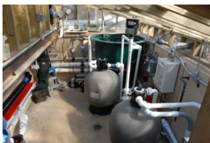
A tour of the filter room
